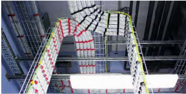
Proper vertical riser installation
